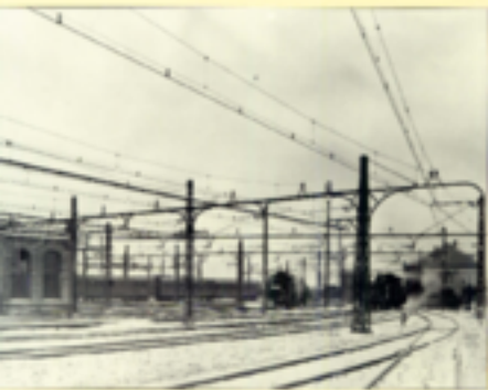
View of the railway yard from the 1911 perspective. The tracks are arranged in a grid-like pattern, and the overhead power lines are visible above the tracks.
